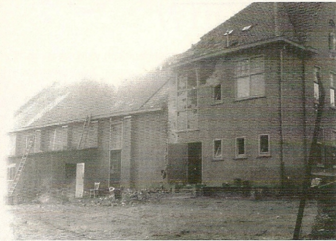
The shelled building.
